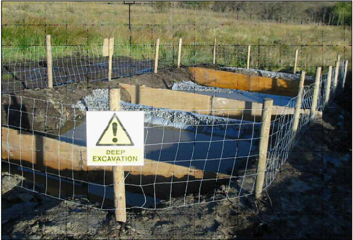
Plate 5.4a: Completed Settlement Pond System
