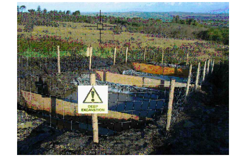
COMPLETED SETTLEMENT POND SYSTEM N.T.SCALE
