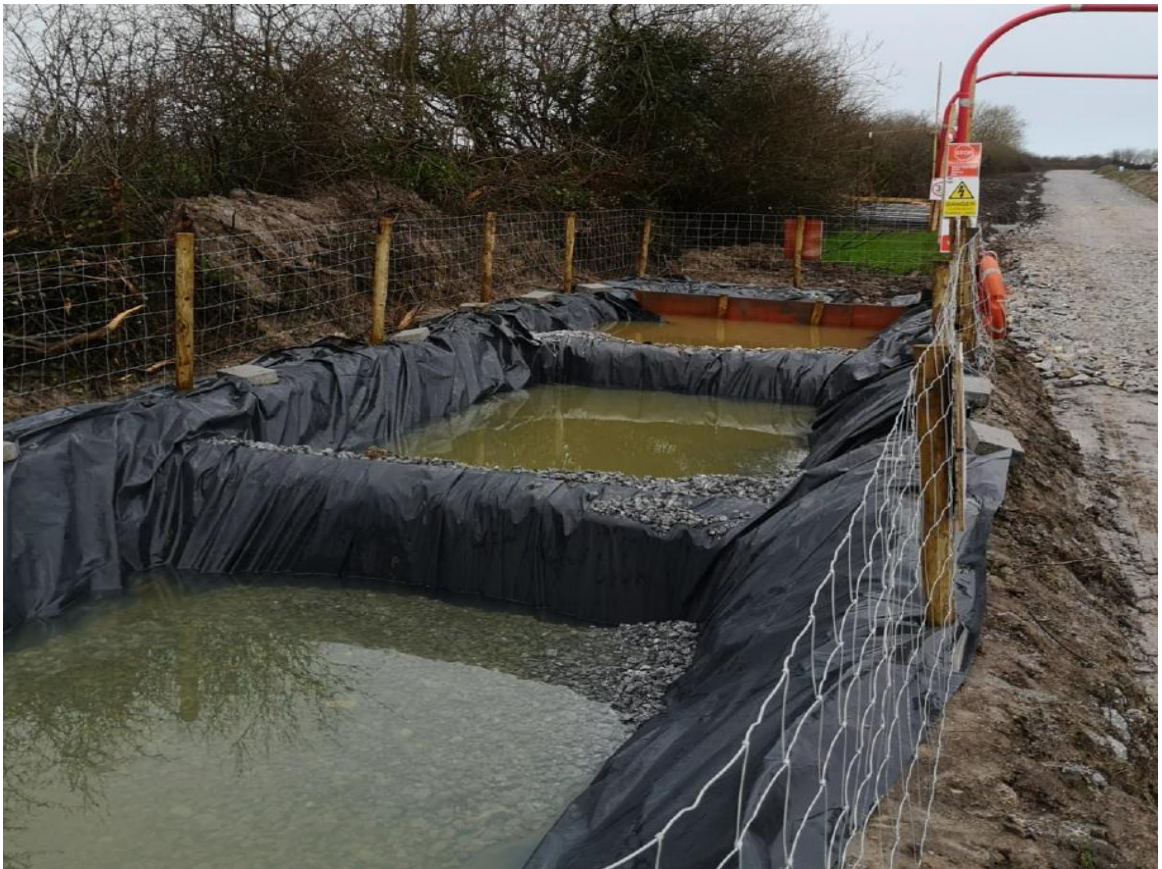
Plate 5.4b: Completed Settlement Pond System Showing Levels of Settlement
